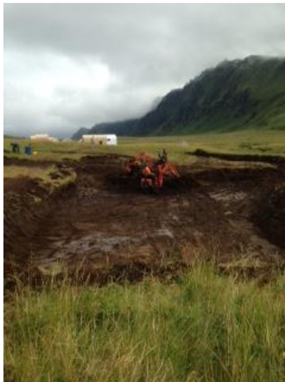
Figure 6: Test sump under construction 5 September 2016.
