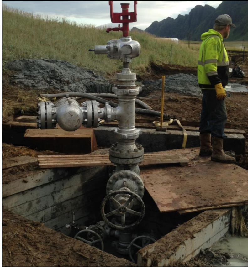
Figure 5: Completed AK-3 wellhead, 7 September 2016.
